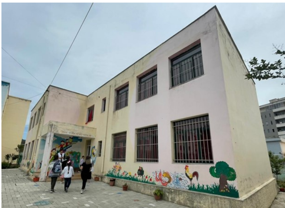
The municipal kindergarten before the intervention
